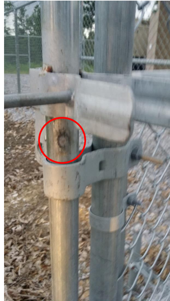
ARC ON GATE POST
