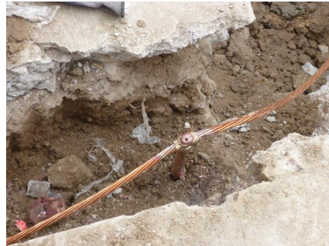
GT CADWELD CONNECTION
