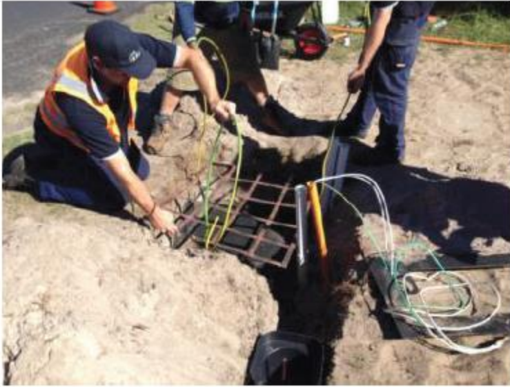
Figure 12 - Install the Earth Mesh
