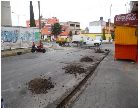
TRENCH TO FEED POWER
