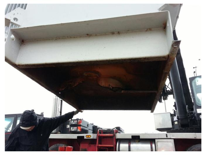
'These photos were from a substation we found where the neutral and tank grounds were stolen from a 3750kva, 34 / 12 kv transformer. We discovered and replaced the grounds not knowing the damage that had occurred under the tank'.
