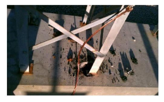
These images were taken of a single phase voltage regulator stand where the regulator neutral and stand grounds were stolen. The stand became energized at line potential and was energized when it was discovered. Voltage/current was seeking ground through the foundation. This was a potentially lethal event.
