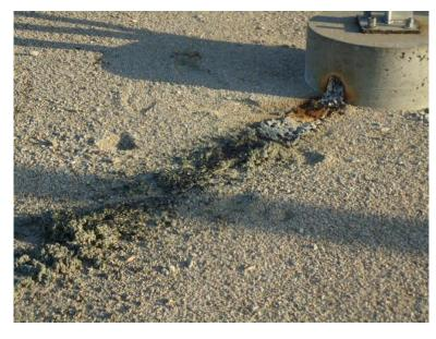
These images are from a 161 kV capacitor bank from which the grounds had been stolen. When the Transmission System Operator energized the ungrounded bank, the structure, including the anchor bolts, became energized. The path to ground was through the foundation
