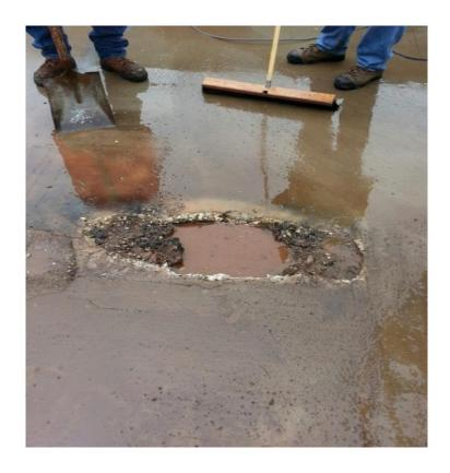
'When the transformer was removed, it was obvious that the current path was attempting to return to the source. The concrete foundation as well as the sub structure of the transformer showed significant damage'.
