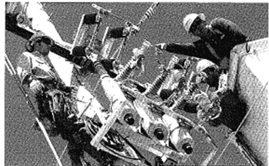
Crews performing the first recloser test install in 2010.
