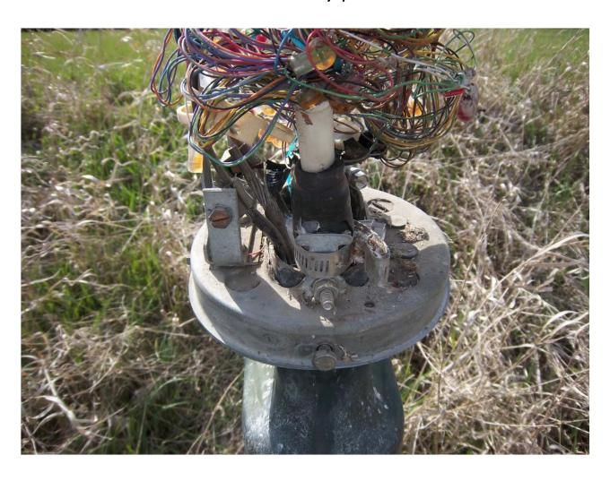
Location on 430<sup>th</sup> Street where 100 feet of cable was replace due to the damage of the existing cable and two wet cable splices.
