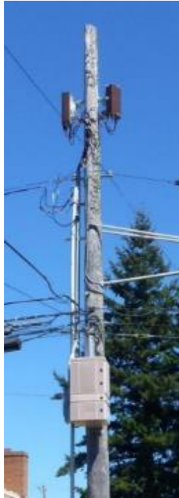
Small Cells on Poles – Notice one on right on same pole as pole mounted utility transformer
