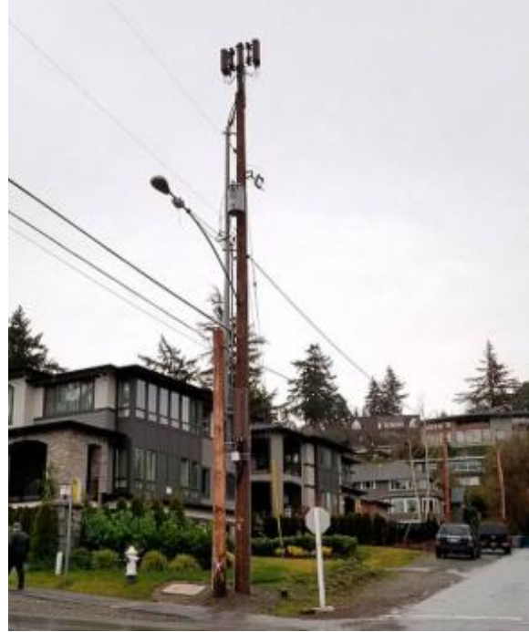
Small Cells on Poles – Notice one on right on same pole as pole mounted utility transformer
