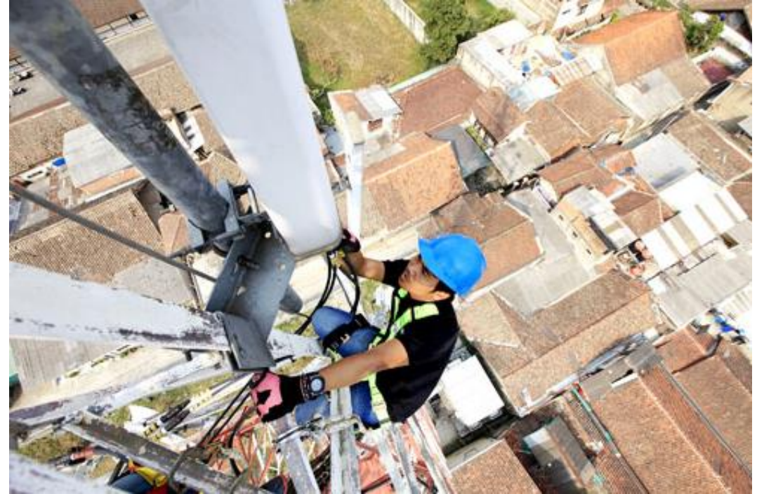
Cell tower in close vicinity to dwellings
