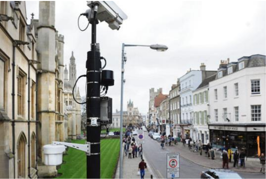
Small Cells on Poles – Notice one on right on same pole as pole mounted utility transformer
