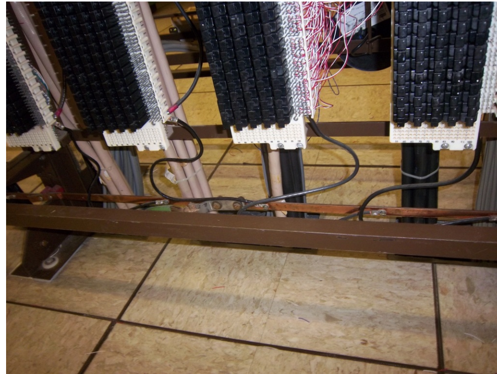
“S” Bends in grounding conductors
