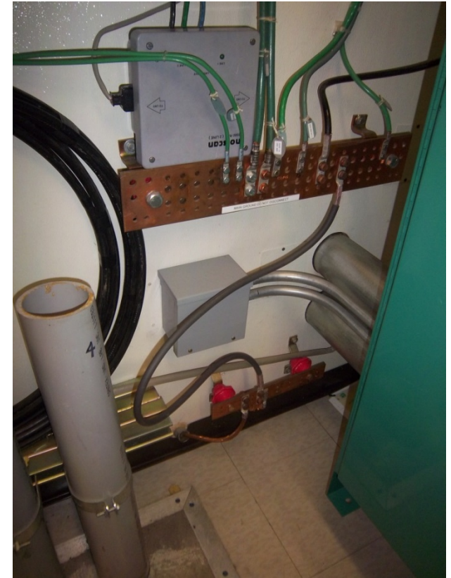
“S” Bends in grounding conductors
