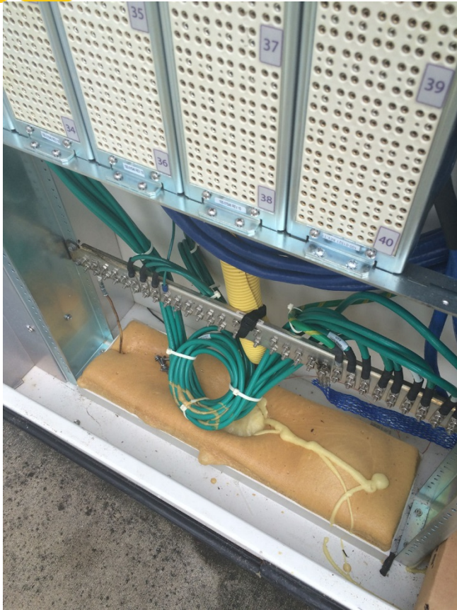
“Inductor” coils in primary protector grounding conductors
