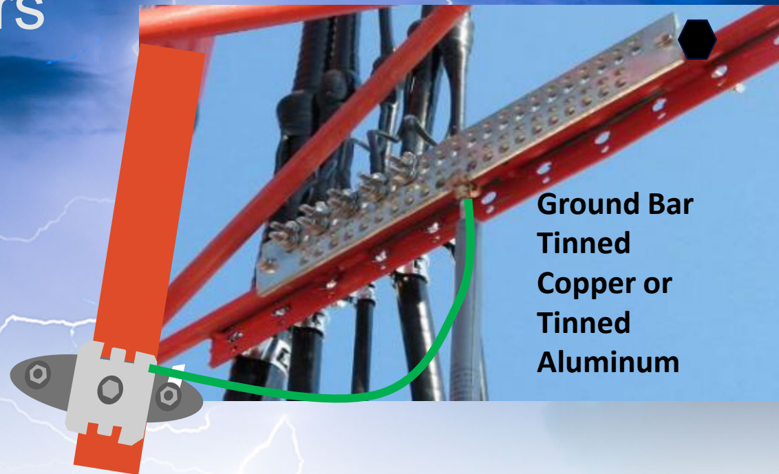
Tower Bonding – Ground Bar & Clamp Details Round Tower Member
