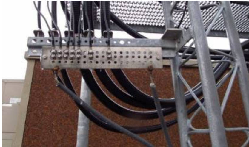
THEFT DETERRENT GROUND BAR MOUNTED ON TOWER CLOSE TO GROUND
