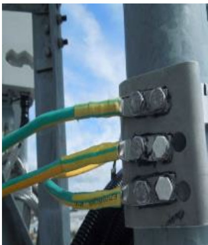
ETMAGS MOUNTED ON RADIO HEAD FRAME, SMALL CELL OR ANTENNA MOUNT
