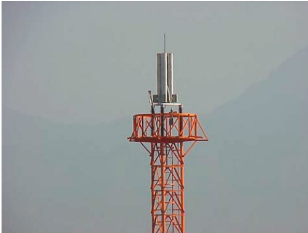
Fig.3 - Tower top with rocket platform
