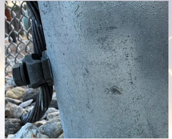
Bare copper connector designed for flat surface on a round steel pipe,
